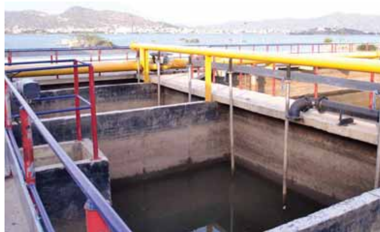
13-MLD-capacity sewerage treatment plant project on Anasagar Lake in Ajmer
