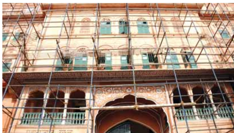
Façade restoration work in progress in Jaipur
